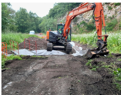
Installation drain grande carrière
